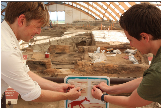
Figure 24. Ian and Izzy finish the installation of a new family trail panel at the entrance to the North Area.
