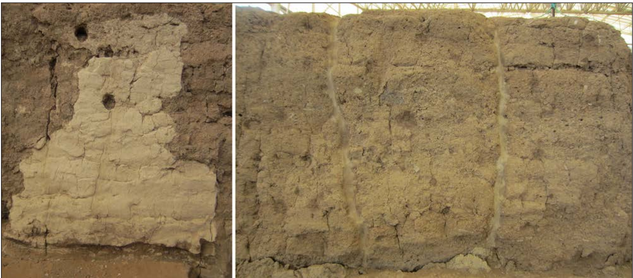
Figure 15.3. Gap fills in B.119, North Shelter. (Left) Plaster filled with Lime/Perlite mixture; (Right) Mudbrick filled with Lime/Perlites mixture.
