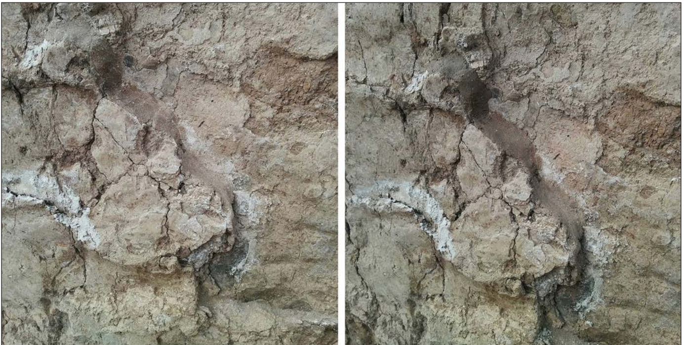
Figure 15.5. Lime/Perlite backings for delaminating plaster in B.132 (North Shelter). Shows drastic colour change in high heat only one hour after application (right).
