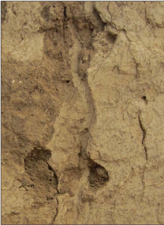
Figure 15.4. Lime/Perlite fill in B.119 showing the formation of hairline fractures during curing.
