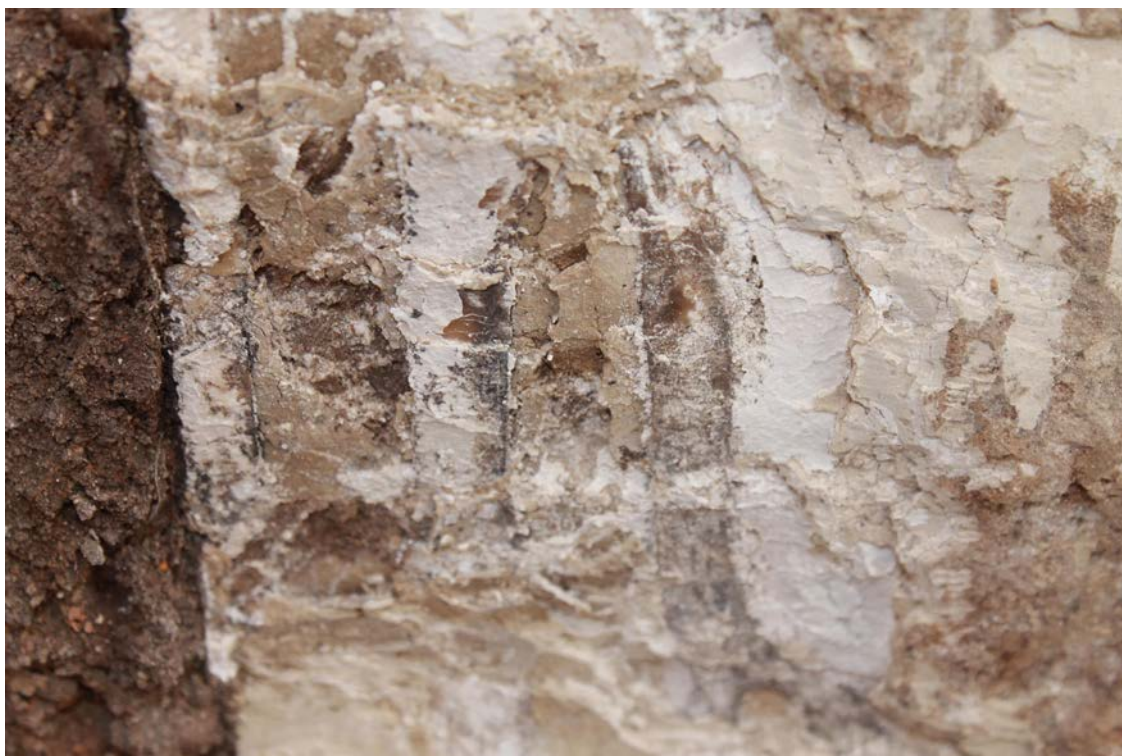
Figure 15.8. Brown colored binder underlying plaster detail.
