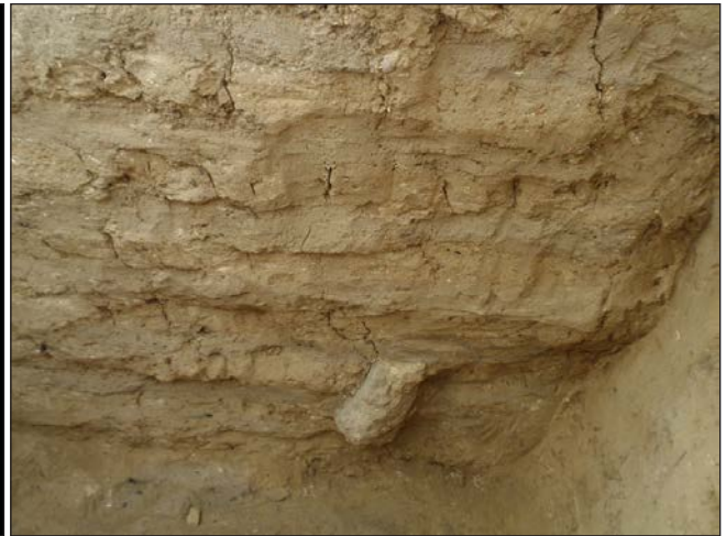
Figure 11.4. The location of quern 20892.x1 in the foundation wall F.8003 (in the photo the courses of mudbricks and mortar are visible) (Photo: Christina Tsoraki).
