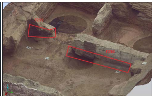
Fig. 21.5. Visualization of wall undercutting in F.230 and F.231 in B.5 due to erosion.
