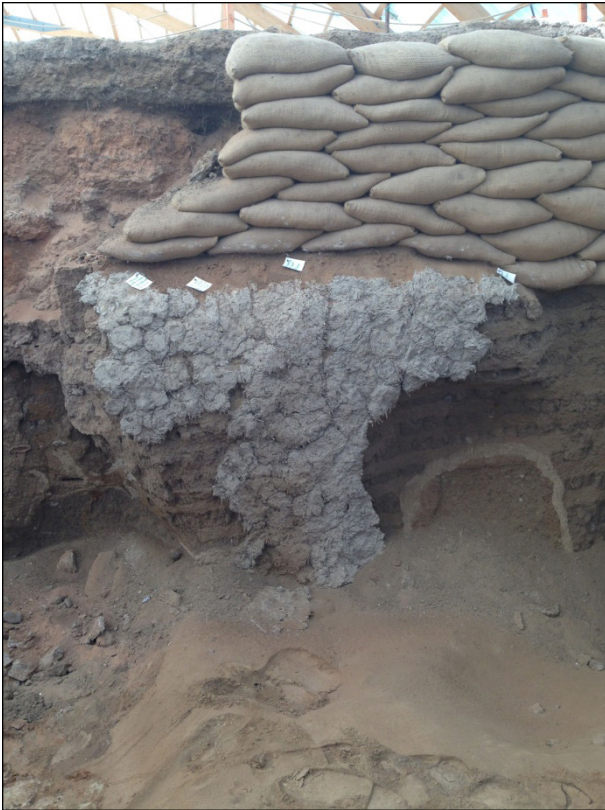
Figure 14.2. Capping experiments from the 2013 season on the south wall of B.5.
