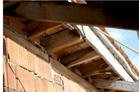
Figure 149. Exposed rafters at eaves.
